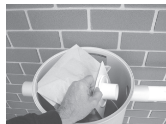
Firmly insert bag into side of unit
