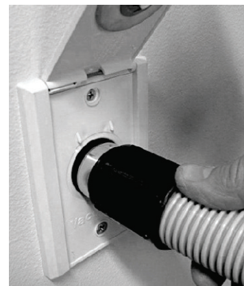
Plug in cuff end of hose into inlet point to activate unit.
